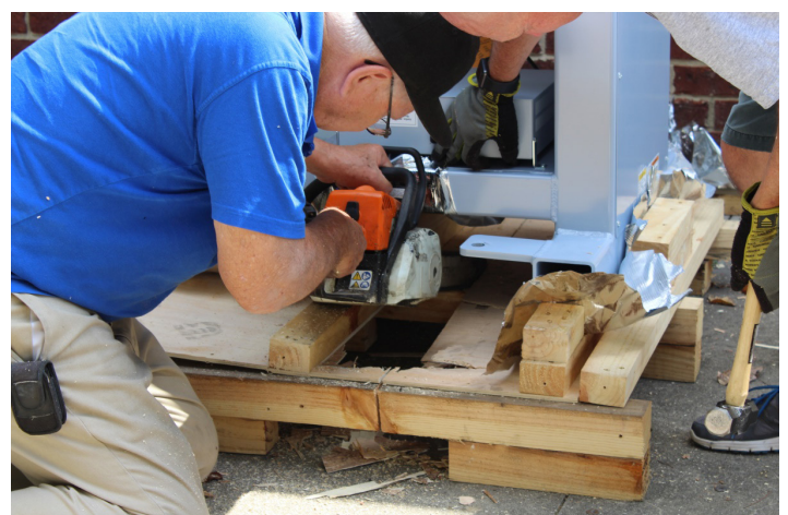
12. In this instance, a chainsaw was used. Be careful not to hit the machine frame with the saw.
